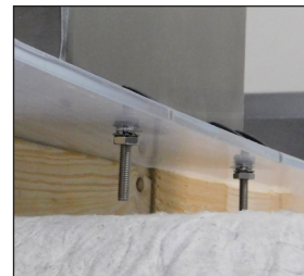
Installed Hardware (View 2)
